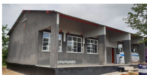
Chipapa Secondary School in Lusaka Province was constructed by Absa Banl in partnership with World Vision
