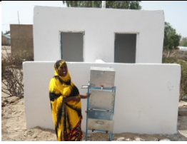
Anisa stands near the latrines constructed for ten H/Hs including her family
