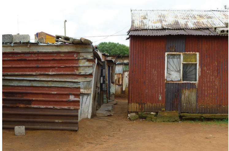
Informal and unsafe housing construction. Orlando East, South Africa.
