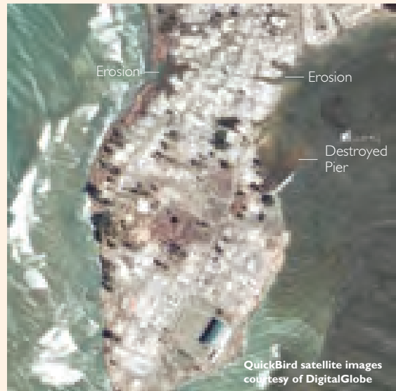
■ Meulaboh, Indonesia: (150 kilometres from epicentre) The images show a small peninsula before (18 May 2004) and after (7 January 2005) the tsunami destroyed many houses
