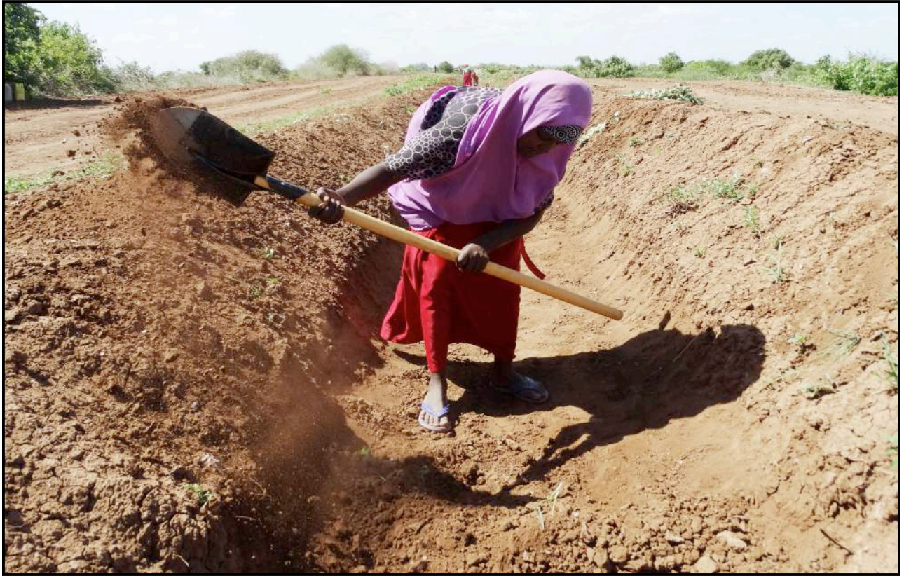
Fama Hussein Shiqow engaging on cash for work canal rehabilitation
