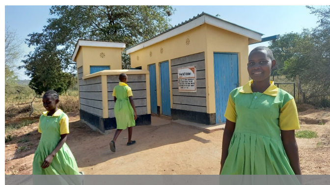
Students at Kavoo Primary School use their new ventilated improved pit latrine, equipped for menstrual hygiene management, along with facilities for handwashing.
