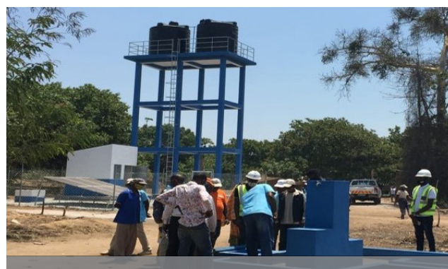
World Vision constructs water systems to provide communities with clean water that is safe for their families.
