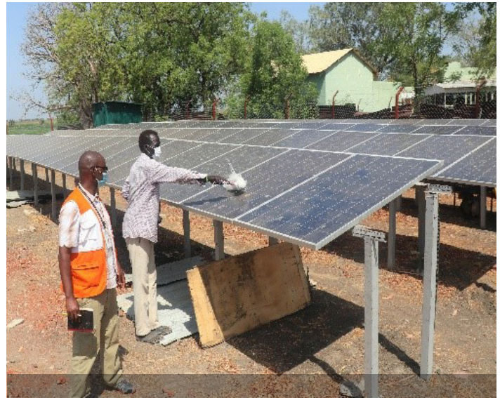
The water operator at the Malakal water system cleans solar panels.
