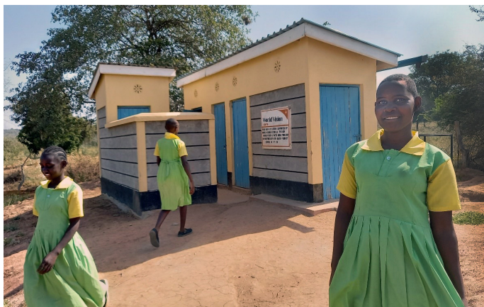
Students in Kenya use their new ventilated improved pit latrine, equipped with space for menstrual hygiene management and facilities for handwashing.
