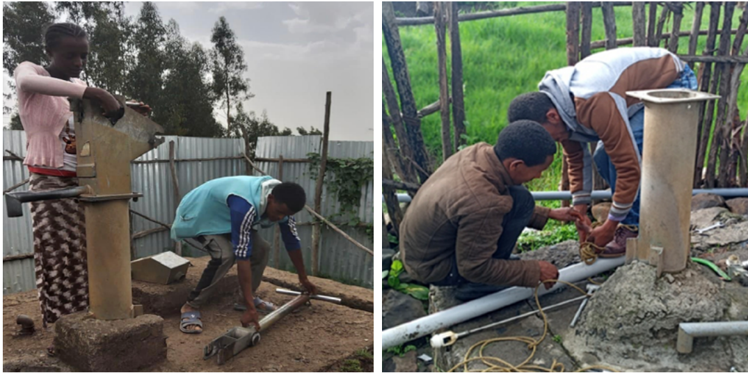
FIGURE 2. Endalek Worku and local entrepreneurs trained by SPIR maintaining a community water supply point.
