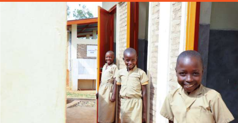
At Cumba basic school, WVIB built a block of latrines children were in need of and that improved their learning environment
