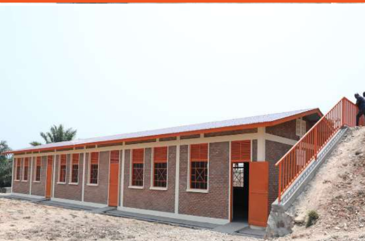
WVIB has constructed 3 classrooms at Ruzibura Basic School in Musigati commune
