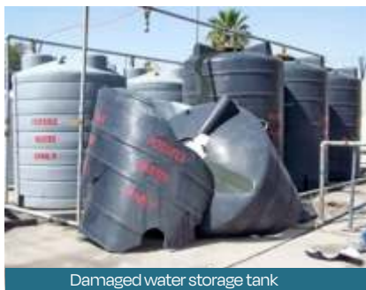
Damaged water storage tank
