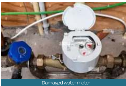
Damaged water meter
