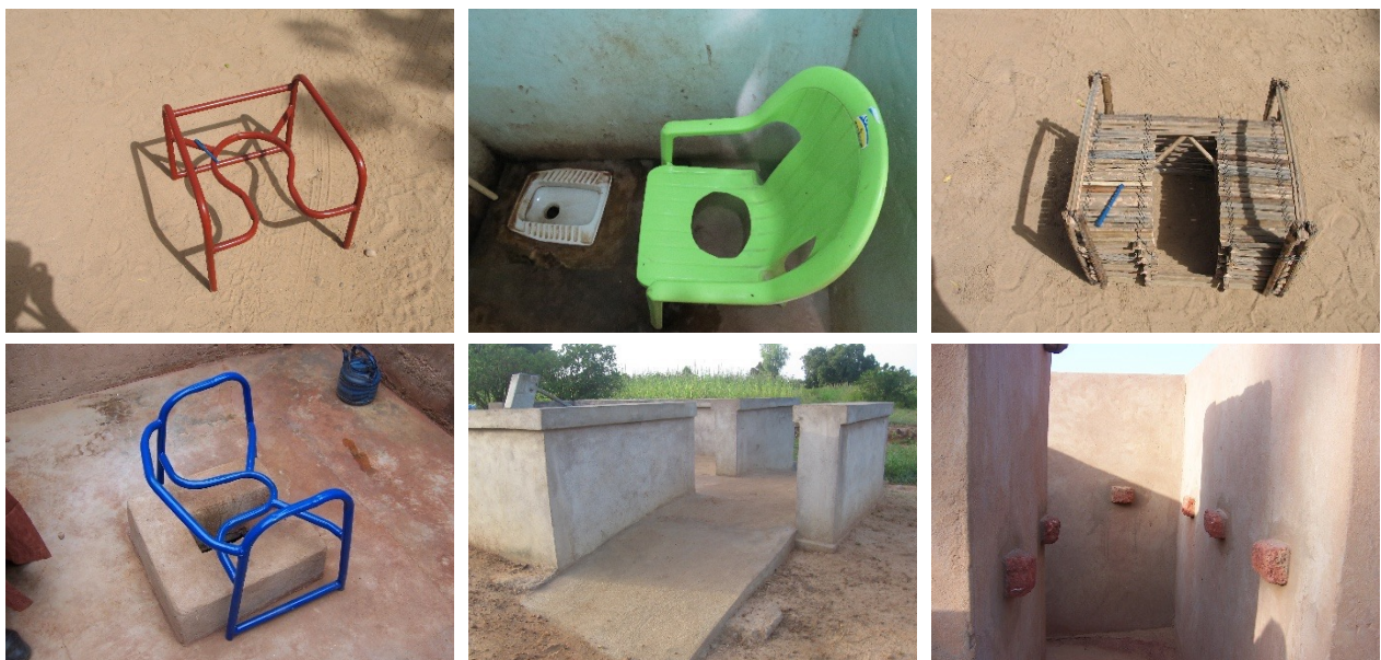
Figure 3. Examples of latrine seats, water point ramps, and improvised brick handrails from disability project in Mali (see Appendix E1 )
