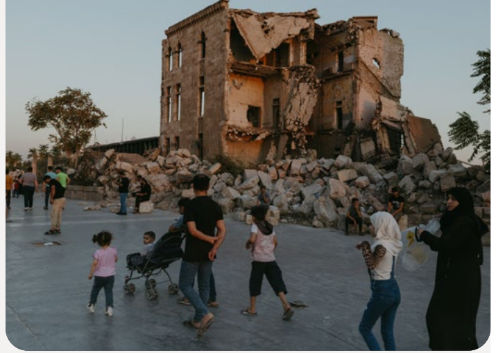
Damaged buildings in Aleppo, Syria, reflect the ongoing impact of conflict on communities.
