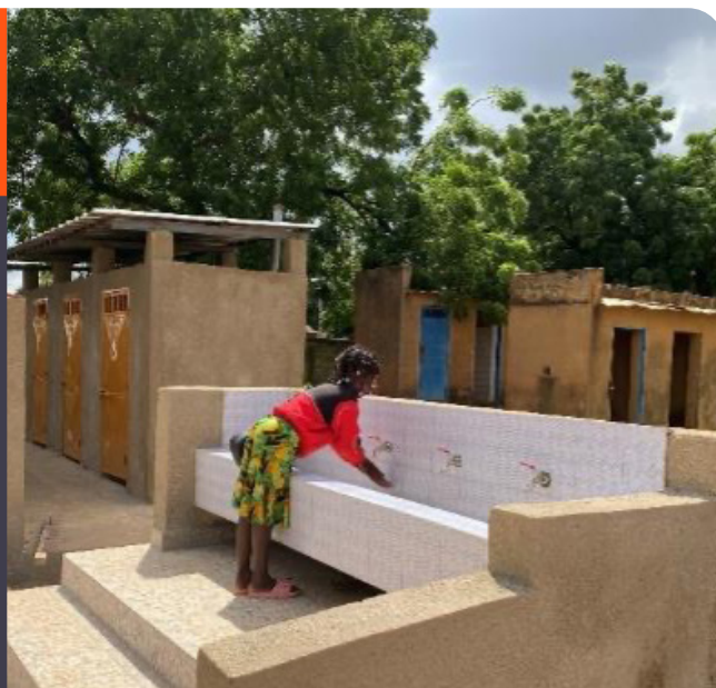
Handwashing stations built at the Somgande primary school, reaching over 1,000 students.
