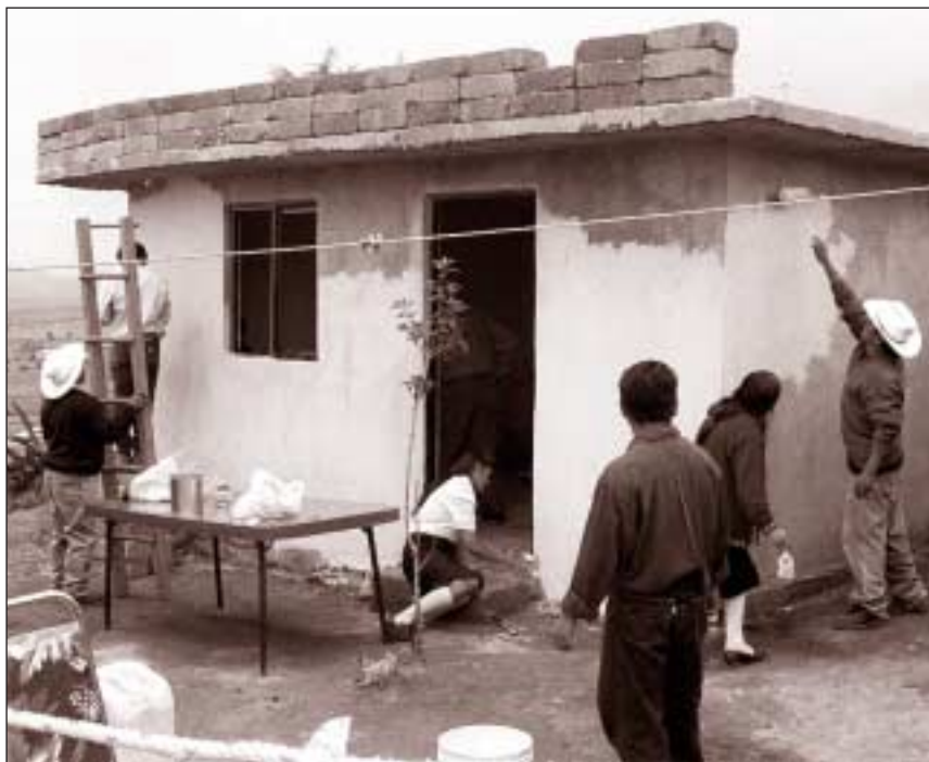
Painting a new brick and cement home in Mazahuas de Choteje, Mexico
