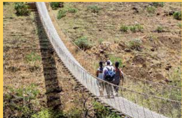
Suspension bridge over the Rib River helped to avert flood threats
