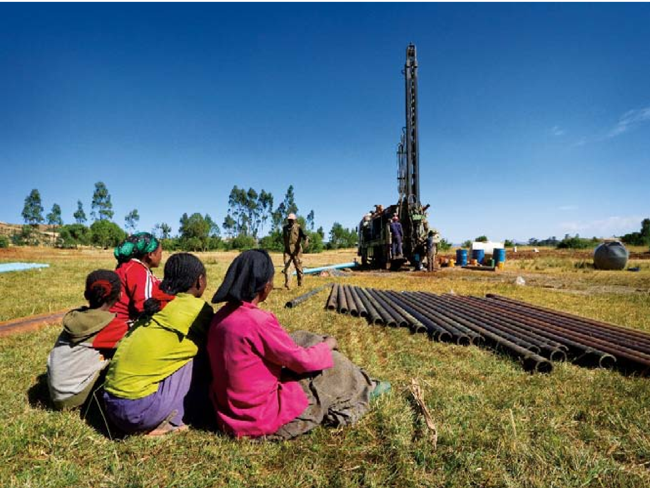
Merawi Ayalew, chief driller for the World Vision contractor that is developing the Dae Wandimtu deep borehole in Wonchi woreda (district) flushes the borehole after drilling it to the required depth.
