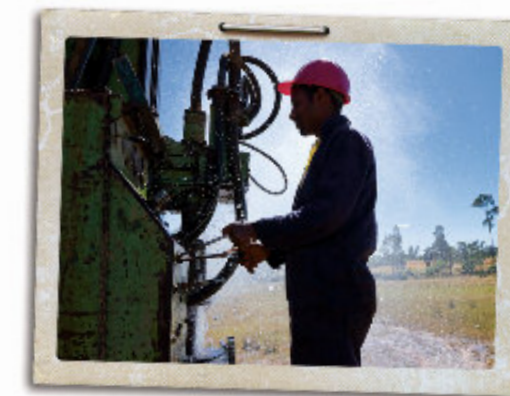
Merawi Ayalew, chief driller for the World Vision contractor that is developing the Dae Wandimtu deep borehole in Wonchi woreda (district) flushes the borehole after drilling it to the required depth.
