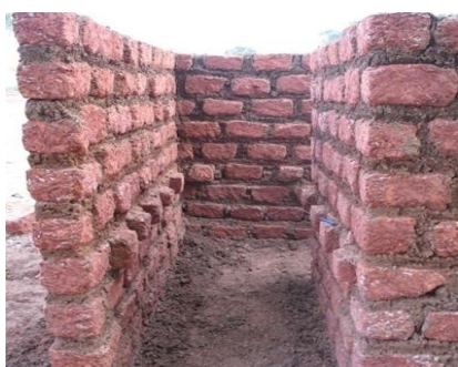
Photograph 1. Latrine handhold supports
