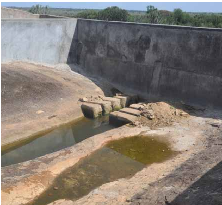
Water harvesting facility - Rock Catchment constructed under NUSAF II Project
