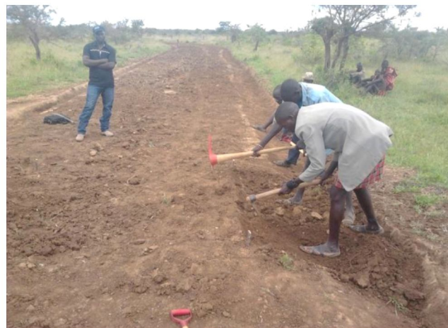
NUSAF II Food for works beneficiaries doing road construction in Kotido District Abim Food Security and Livelihoods Project (AFWASH)
