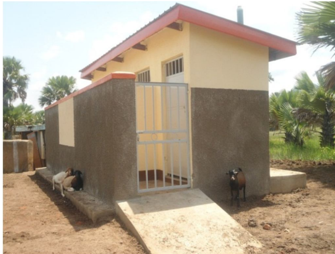
VIP Latrine constructed in Pupukamuya Primary School with USAID funding.
