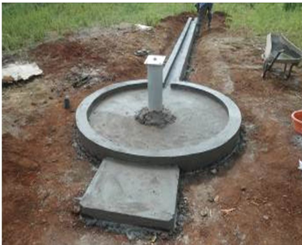
Borehole construction being conducted in Abim under the AFWASH project.
