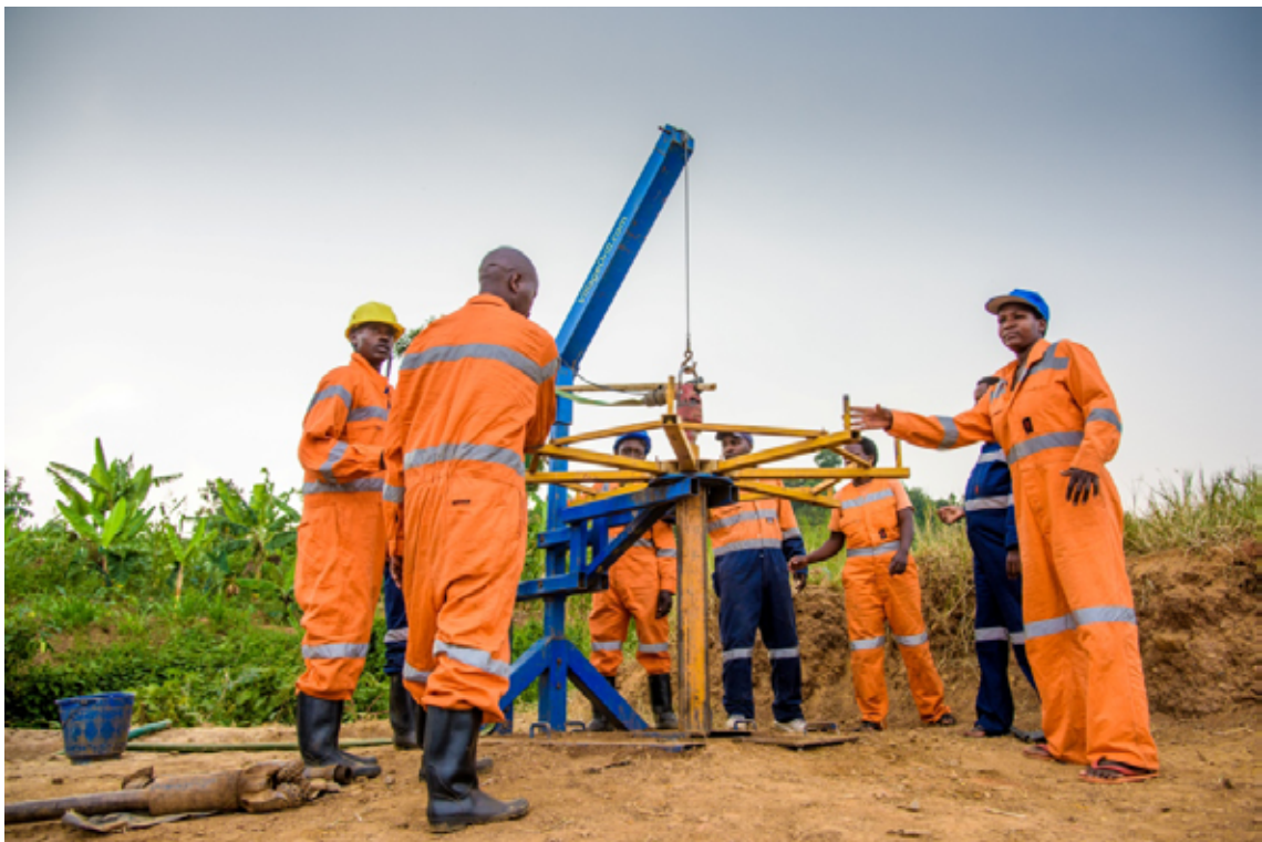
Cooperative members trained by World Vision drill new boreholes using the Manual Drilling Technology.
