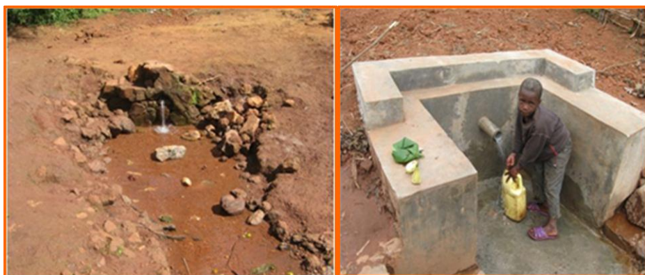
Bitambwe Spring, before and after rehabilitation, Gashoho
