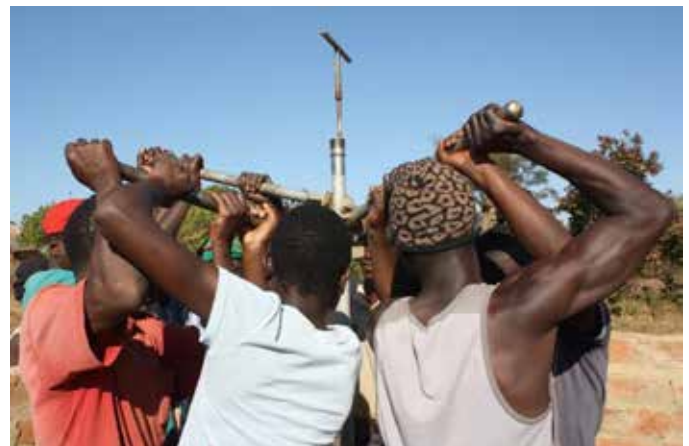
Borehole rehabilitation in Zambia.
